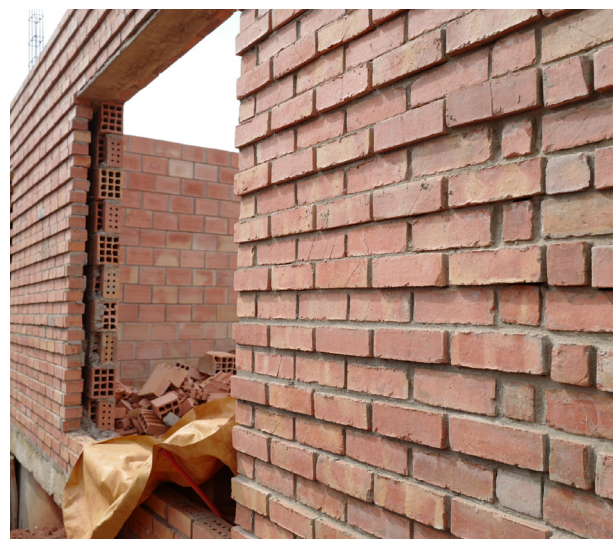
Figure 52. Carre Hinnoudo construction site
