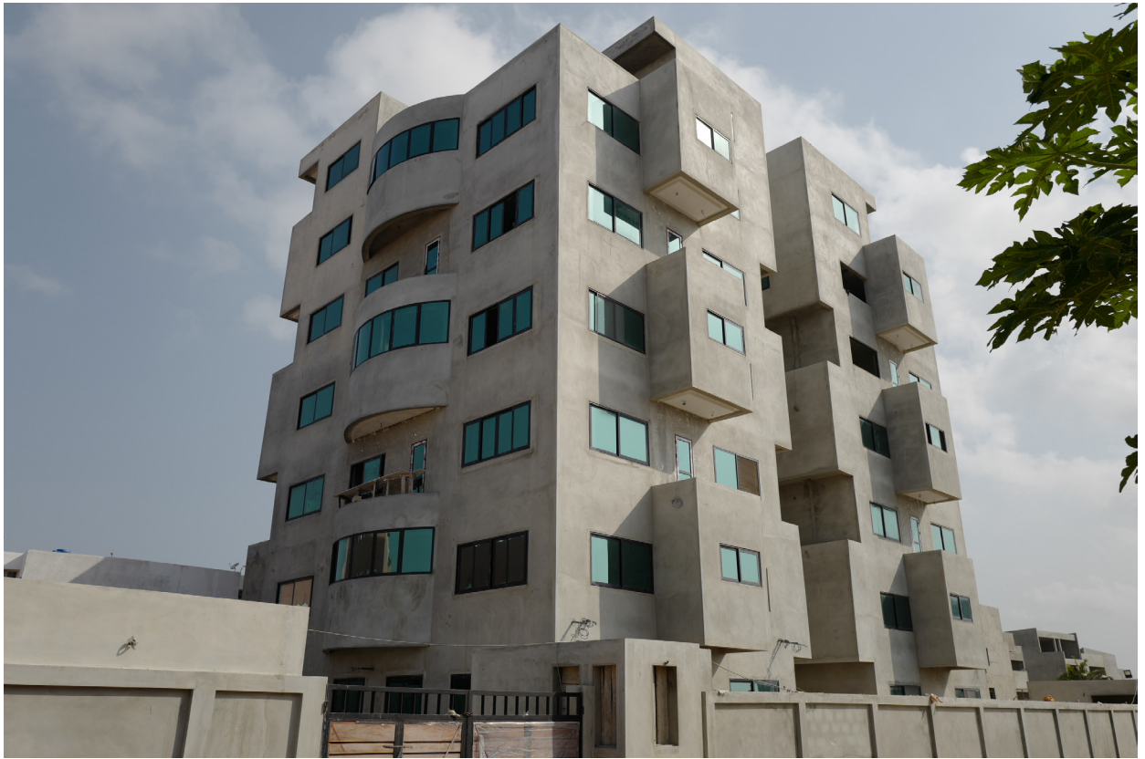
Figure 24a. Concrete under construction in Cotonou
