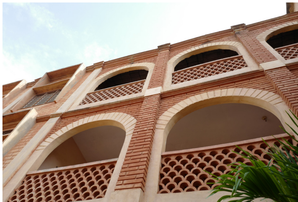
Figure 28a. CEB construction company Art Deco
