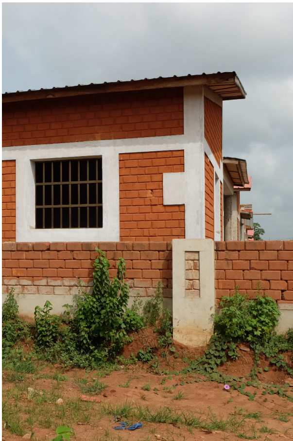
Figure 21. Reinforced concrete skeleton
