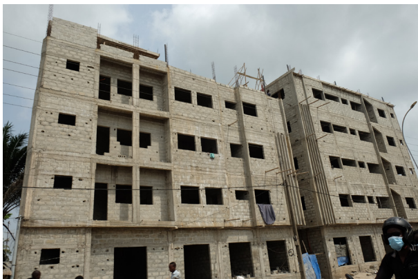
Figure 24d. Concrete under construction in Cotonou
