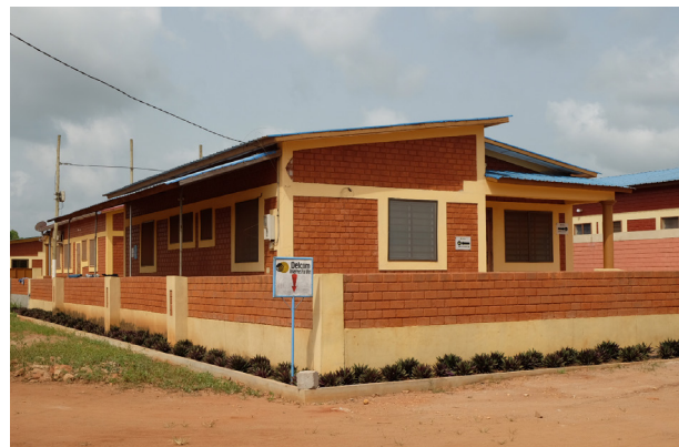
Figure 29b. Cite Bethel, CEB construction
