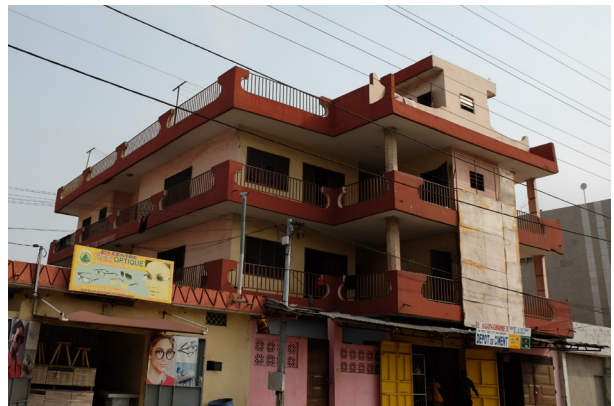
Figure 23c. Concrete housing in Cotonou
