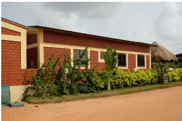
Figure 29a. Cite Bethel, CEB construction
