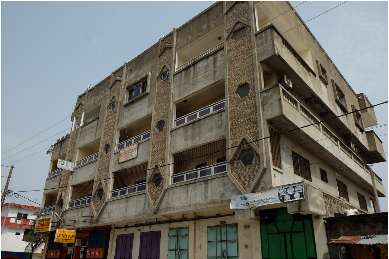
Figure 23a. Concrete housing in Cotonou
