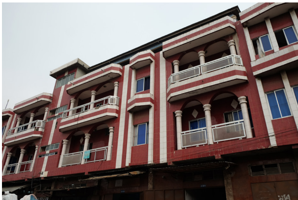
Figure 23b. Concrete housing in Cotonou
