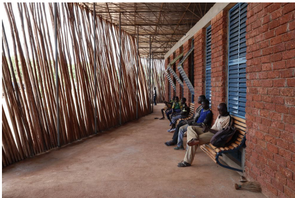
Figure 40. Schorge secondary school in Gando
