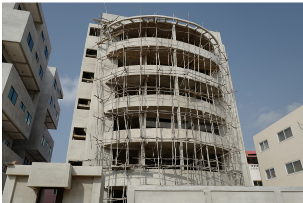
Figure 24b. Concrete under construction in Cotonou
