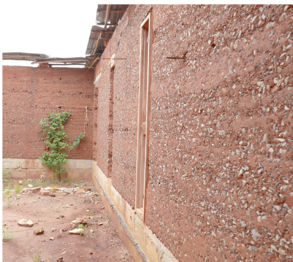
Figure 51. Carre Hinnoudo construction site
