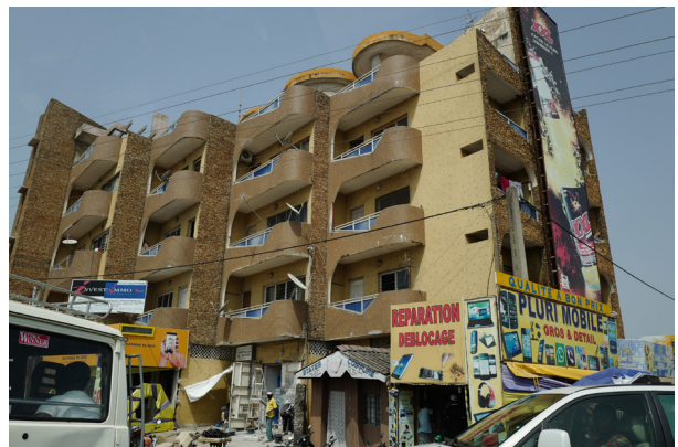
Figure 23e. Concrete housing in Cotonou
