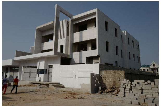
Figure 24c. Concrete under construction in Cotonou
