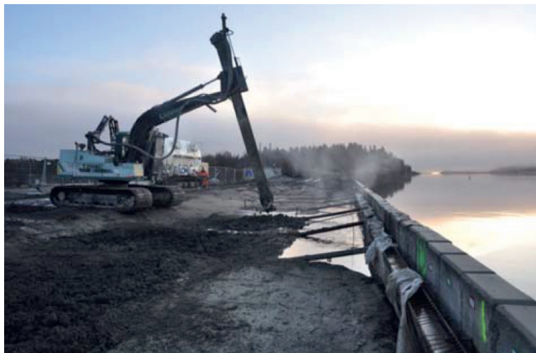
Mass stabilisation of dredged contaminated sediment behind concrete quay wall
