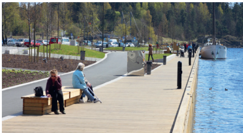
Completed project – stabilized sediments form new quay wall and walkway
