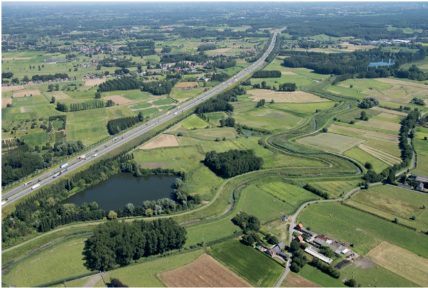
Figure 1. Project area seen from the south
