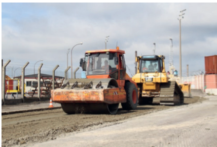
Leveling and compaction of the sub base road layer
