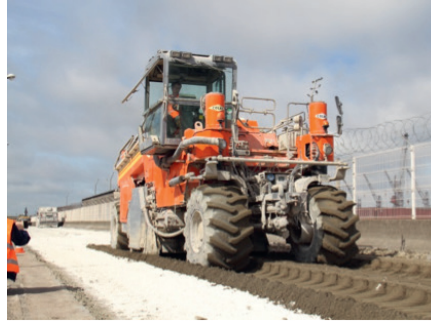
Pre-treated sediments used in sub base road layers (left) and application of hydraulic binders (right)
