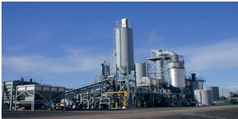
Figure 2. Cement-Lock Demonstration Plant , Bayonne, New Jersey
