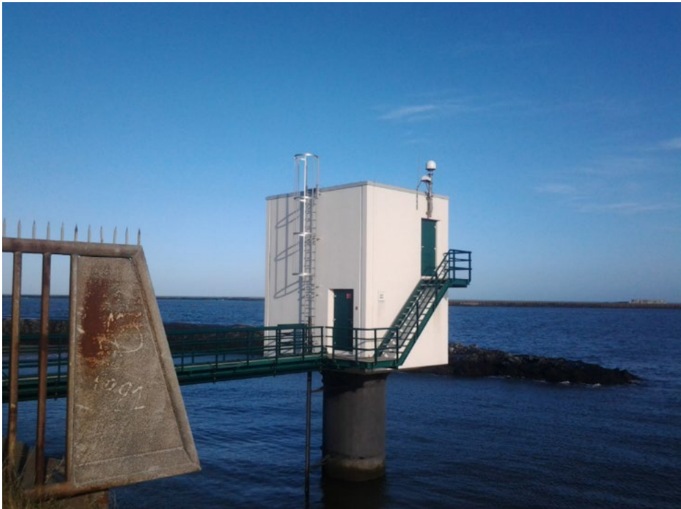
Figure 4-4: LMW Measurement Station (RWS, 2017)
