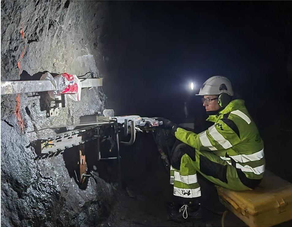
**Figure 3.17:** The sawing of the slot of the flatjack (by Jeras Dieleman).
