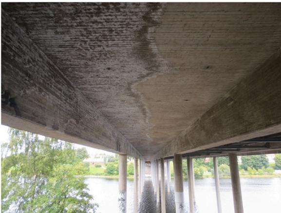
Fig. 12. Signs of water penetration of the bridge deck in outermost region of the bridge. Image courtesy of Dr. Ing. A. Aas-Jakobsen AS.
