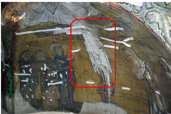
Fig. 3 Detachment of wall-mosaics from a masonry wall due to bulging of the mortar layer because of compression forces within the layers, Monastery of Chios (1045–1056 A.D.), Greece. Photo archive: Lab of Building Materials AUTH
