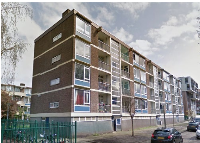
Figure 5.2: Street view of case study building (google maps)
