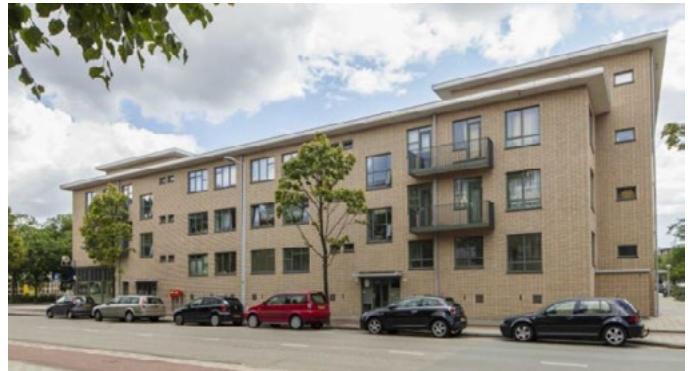
Figure 2.5: Image of Lucellestraat from main street view pre (image above) and post retrofit (image below).
