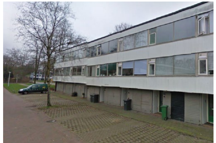
Figure 2.6: Image of Siboldustraat from street view pre (image above) and post retrofit (image below).
