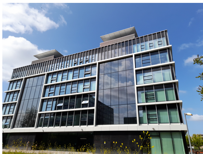
Figure 3: In the Langeveld building, a multipurpose study centre, at the Erasmus university in Rotterdam, a very low pressure hybrid ventilated building with solar/wind towers still has openable windows. The air can be cooled and humidified via a droplet shower in the central shafts, creating significant air pressure to induce the air flow [6,7].
