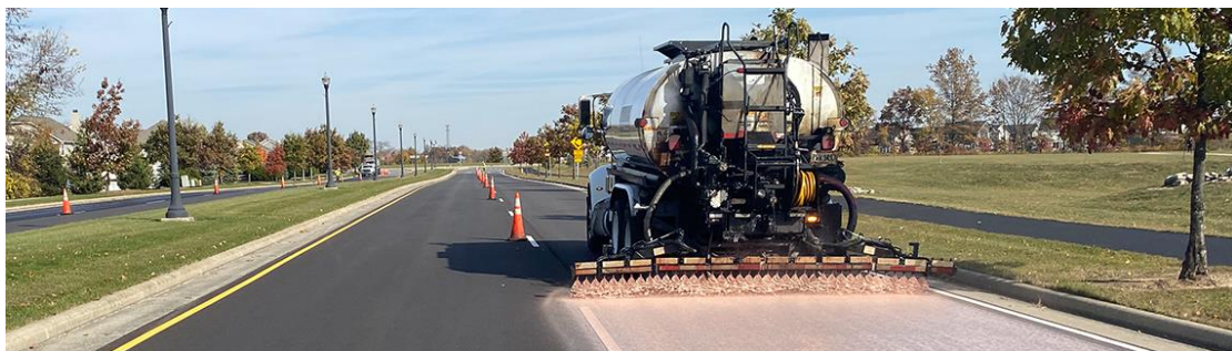
Figure 4-4 A sprayer spraying rejuvenator on the road (Pavement Technology, n.d.)
