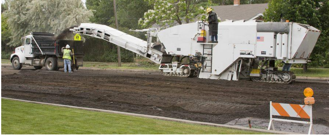
Figure 4-2 Pavement milling (Walkos, 2020)
