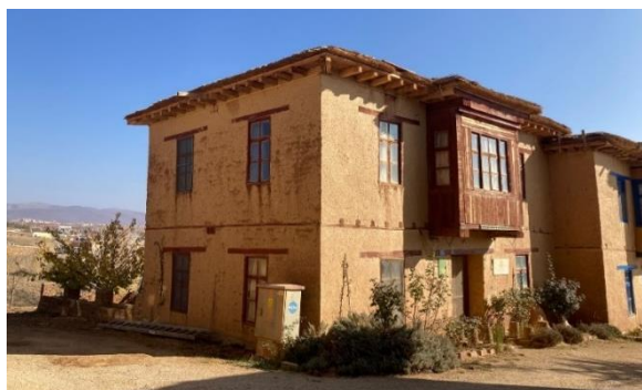
Figure 2: Contemporary example of historically built 2-story high mudbrick house in Sonsuz Şükran. (Own image, 2021)
