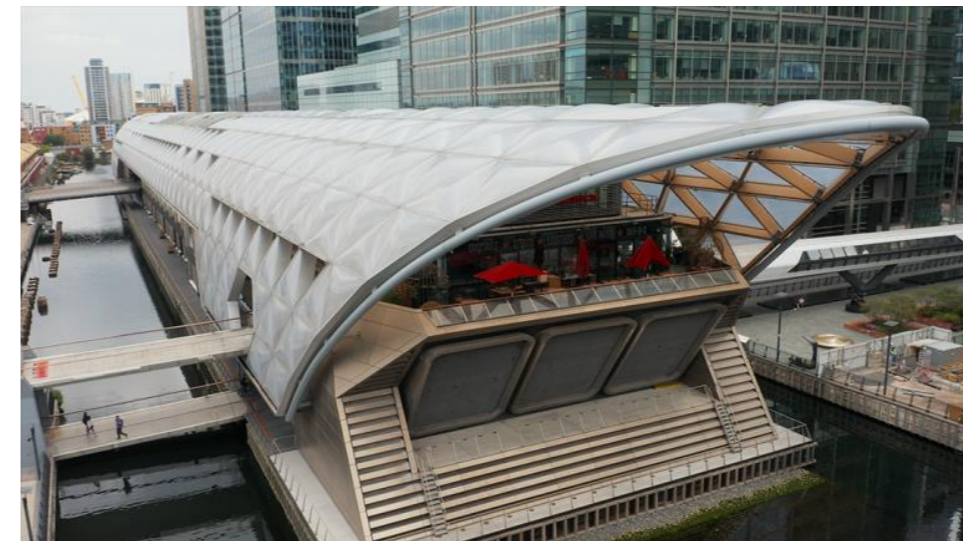
Figure 2. Image of the canopy of the project
