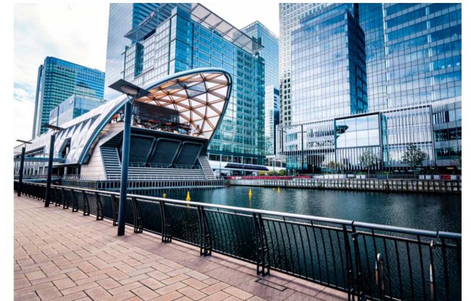
Figure 41. View of the building from one of its sides on the adjacent river.
