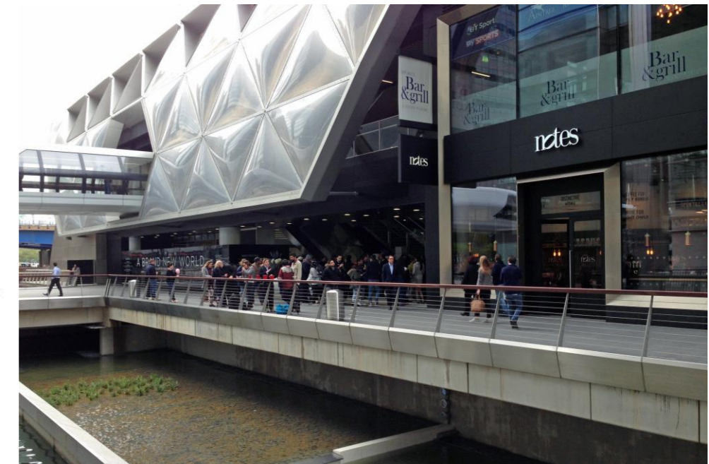
Figure 46. The places of the water storages on the both sides of the building.
