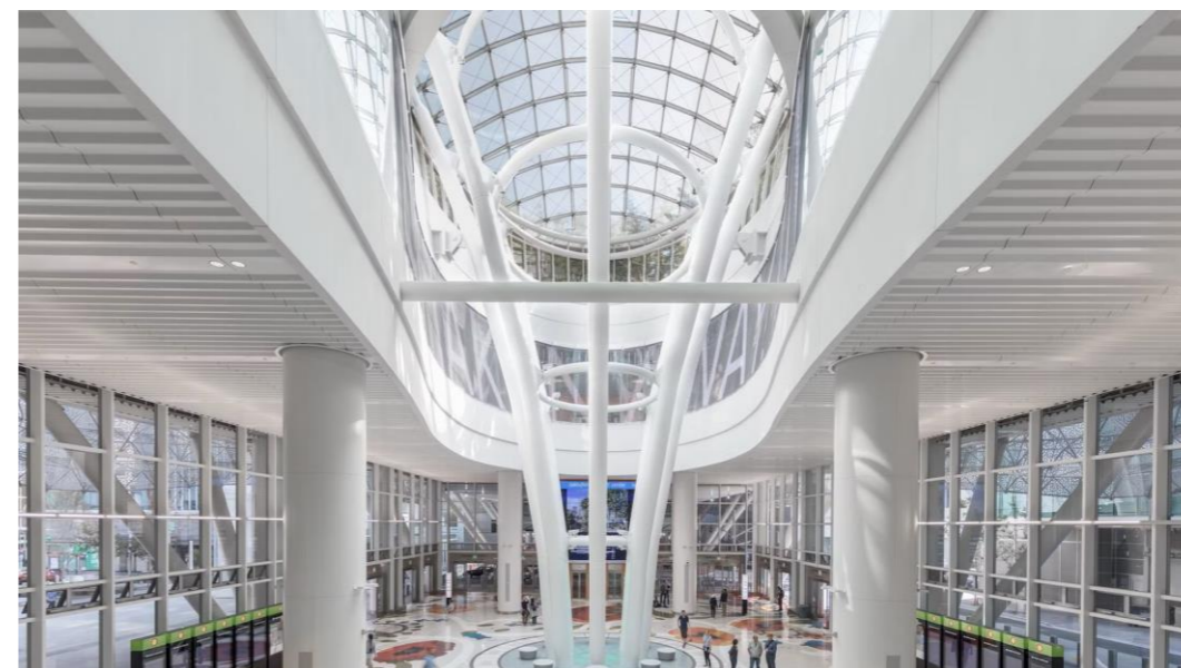
Figure 10. Image of the skylight openings, the light columns.
