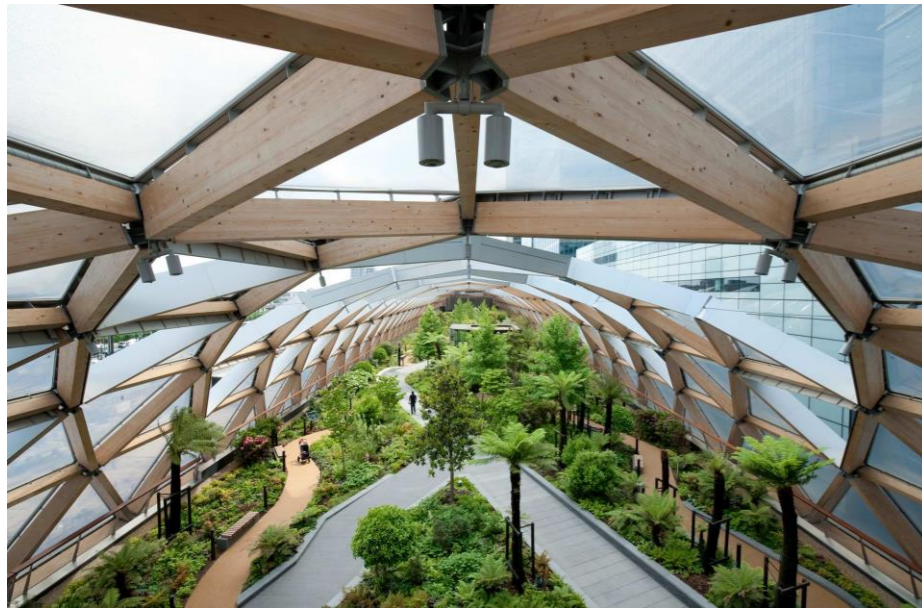
Figure 48. View of the roof garden.
