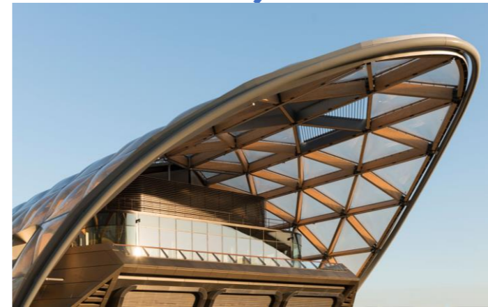
Figure 18. the timber construction of the roof.
