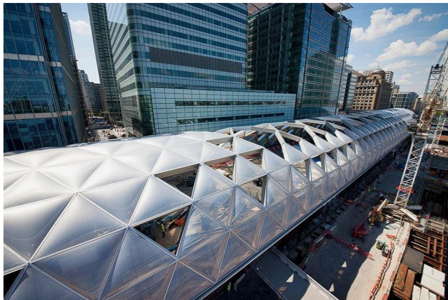
Figure 39. The openings within the canopy of the roof.
