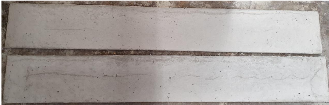
Figure 32 SHCC smooth laminates (the first series of the beams)
