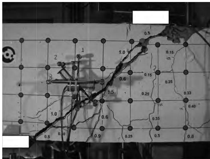
Figure 2 Example of Shear Compression Failure in a reinforced concrete beam [13]
