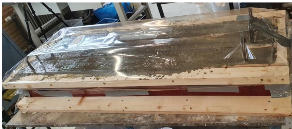
Figure 34 Two hybrid beams and one reference beam sealed (the first series of the beams)
