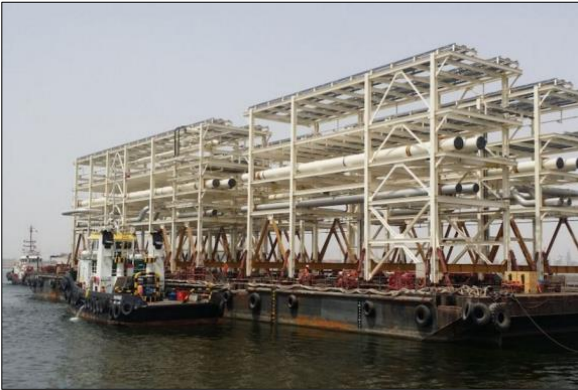
Figure 1-3 Sea transport of pipe racks [3]
