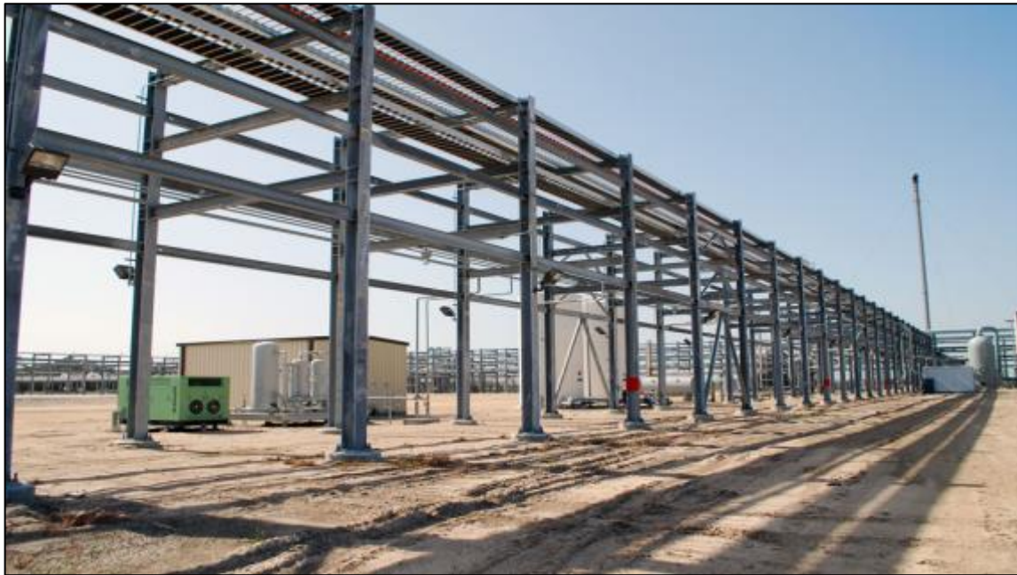
Figure 1-2 Typical example of a pipe rack [2]
