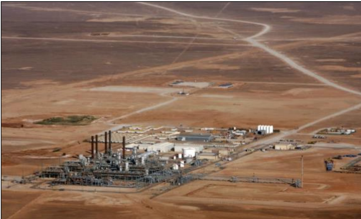
Figure 1-1 Typical example of a pipe rack [1]
