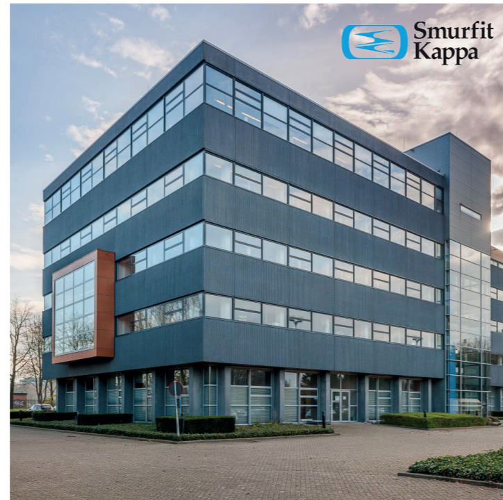
Figure 38 The Smurfit Kappa Experience Centre in Oosterhout, the Netherlands. This is where the meeting was held.
