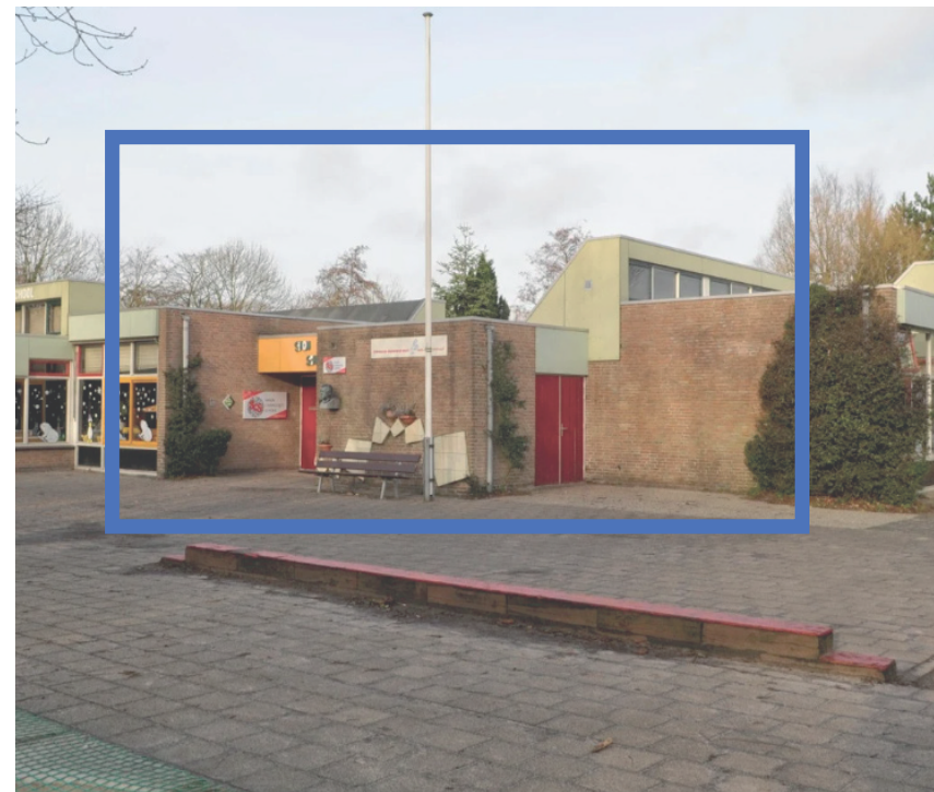
- Ineffective thermal protection
