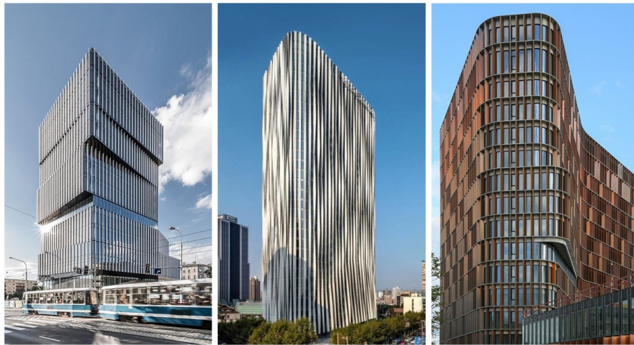
Figure 8.21: : Examples of buildings in Singapore with the integration of vertical shading louvres on the facade. From left to right: Silver Tower Center (Source: https://archello.com/project/silver-tower-center ), Hongkou Soho' office tower (Source: https://www.baunetz.de/meldungen ) and The Maersk Tower (Source: https://architizer.com ).
