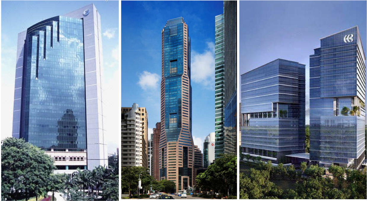
Figure 3.8: Examples of buildings rated with Platinum Award. Revenue House (Source: https://www.streetdirectory.com ), Republic Plaza (Source: http://www.skyscrapercenter.com/building/republic-plaza/635 ) and The Metropolis (Source: http://www.servcorp.com.sg ) (from left to right).
