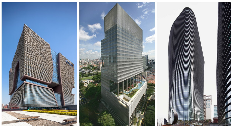
Figure 8.22: : Examples of buildings in Singapore with the integration of horizontal shading louvres on the facade. From left to right: Xi'an Jiaotong-Liverpool University (Source: www.archdaily.com ), One George Street Singapore (Source: https://architizer.com/projects/one-george-street/ ) and Twin Tree Tower (Source: www.archdaily.com ).
