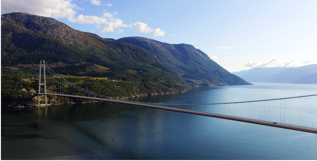
Figure 5: The Hardanger Bridge.
