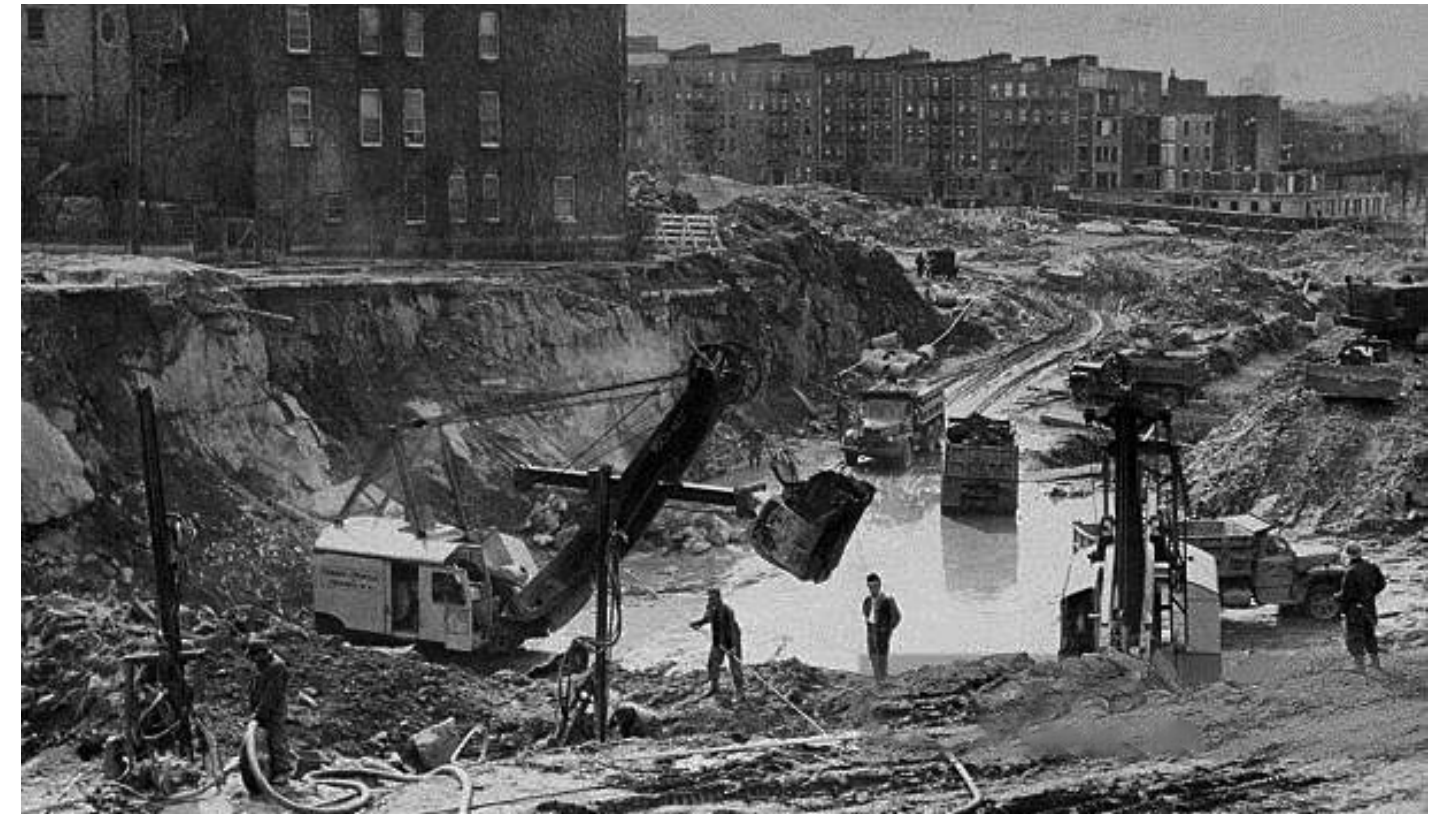
Robert Moses' Cross Bronx Expressway construction, 1948-63.
