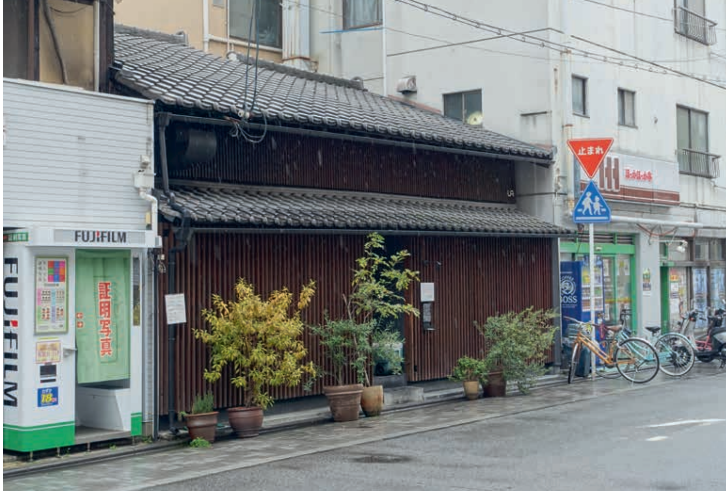
3. Streetscape in Kyoto: a renovated, authentic machiya surrounded by more recent architecture (photo Hielkje Zijlstra, 2015)
