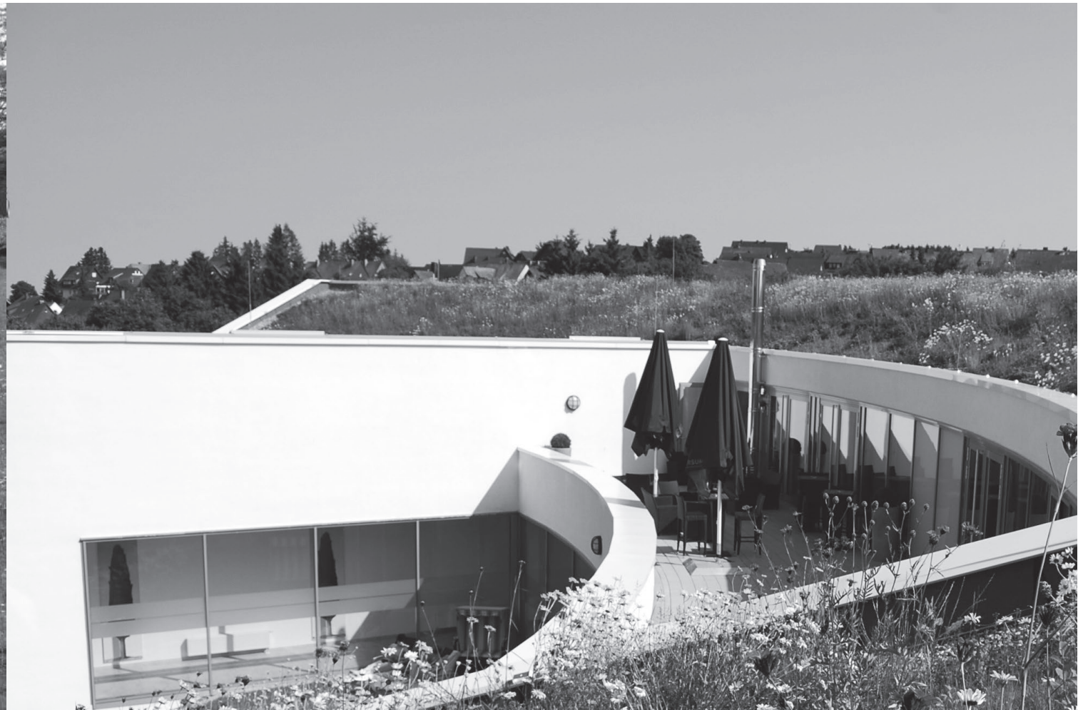
Intensive green roof
