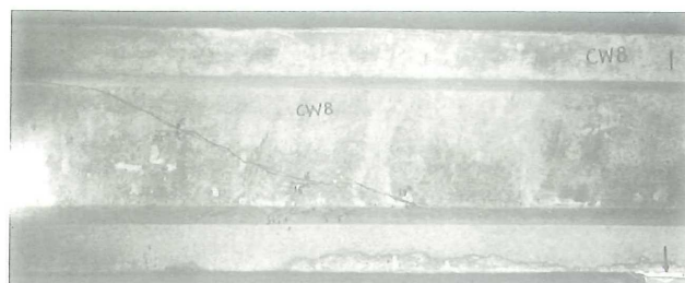
Figure 3.24: Crack pattern CW8[9]
