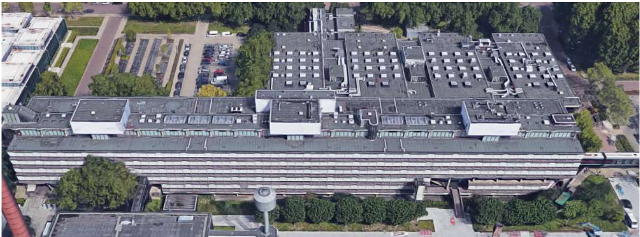
Image 5. Gemini building of the Technical University of Eindhoven. Source: google maps 2019
