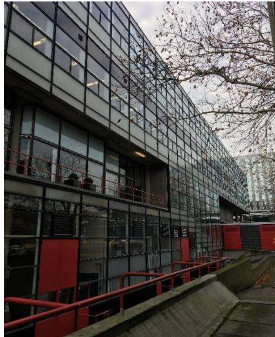
Image 7. North façade of the Gemini south building
