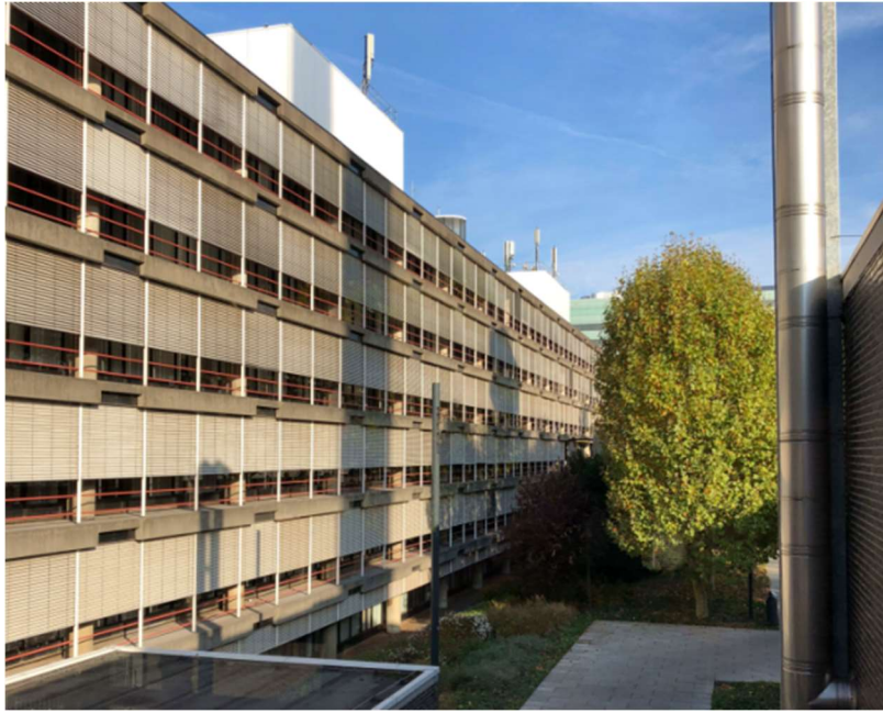
Image 6. South façade of the Gemini south building
