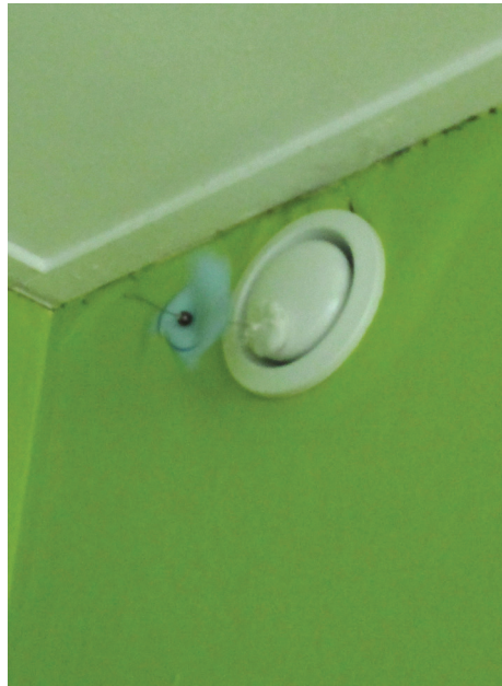
Fig. 72 - The fan is attached by the resident in the single-use evaluation. The fan supports the idea that the system works
