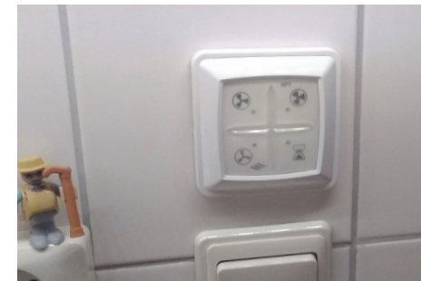
Fig. 20 - Residents of the explorative interview showed this ventilation control. The resident has to select the function suitable for the situation. The control gives no indication of the setting it is currently on.
