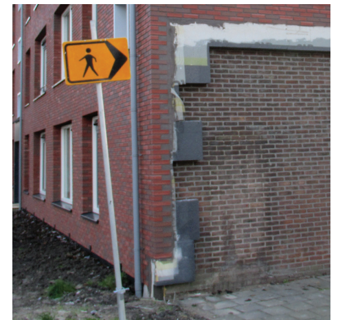
Fig. 4 - One of the 183 zero energy ready units, with the 2ndSKIN insulation clearly visible
