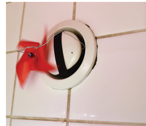
Fig. 66 - Fan attached to extract valve by means of elastic
