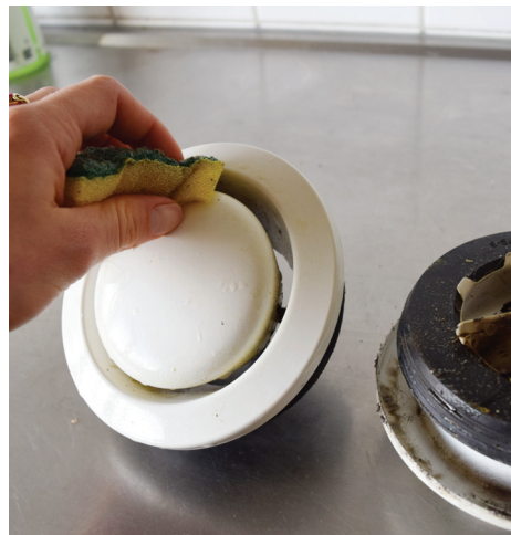
Fig. 26 - Residents are expected to clean the valves, however cleaning the valve without adjusting configuration or mixing valves is a challenge
