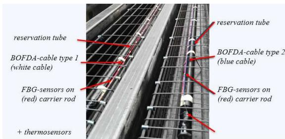
Figure 3. Instrumentation of the pile in formwork
