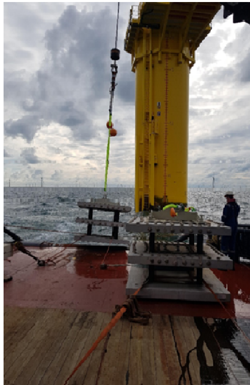
Figure 5.16: The structures have been placed offshore from a multicat vessels
