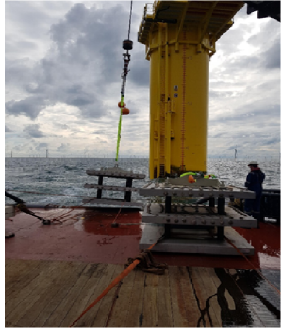
Figure 5.7: The structures being placed off the multicat vessel near the MP
