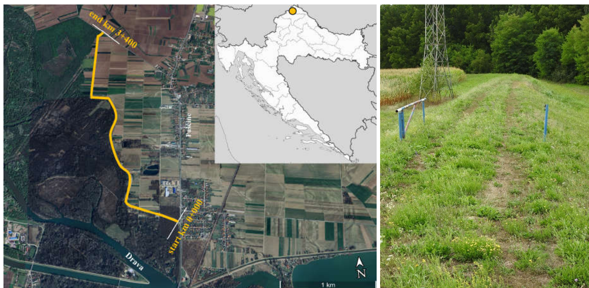
Figure 3. The layout and the current condition of the Pušćine levee
