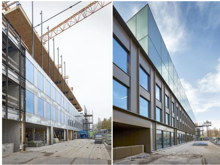
Figure 7-10: EDGE Olympic facade construction (retrieved from van Eesteren, 2021)
