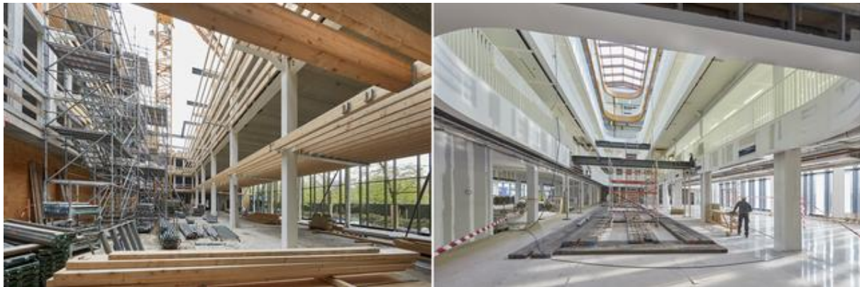
Figure 7-11: EDGE Olympic structure construction (retrieved from van Eesteren, 2021)
