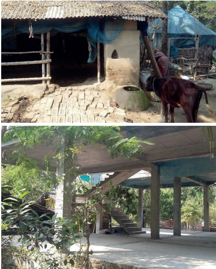
Figure 4.5 Examples of kuccha structures (Top) and pucca multi-level structures under construction (Bottom) in Hogladanga (Photo courtesy Gomes, 2017)
