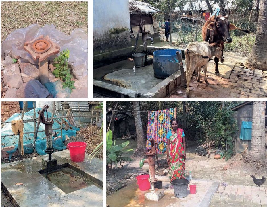
Figure 5.7 (clockwise from left) Private tube wells in Hogladanga: (a) failed private tube-well installations; (b,c,d) operational private tube wells (Photos courtesy Gomes, 2017)
