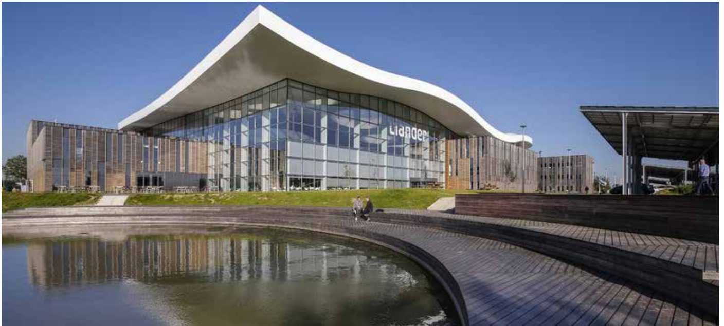
The new office of Alliander, with waterbuffer in front (De ingenieur, 2015)
