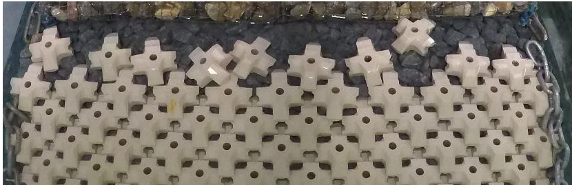
Figure H-51: Test series 1.1.1 Repetition – Before Test with N_s=1.77 (70% design conditions)
