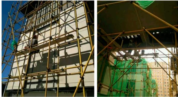
**Figure 12.** The installation process of insulation boards.
