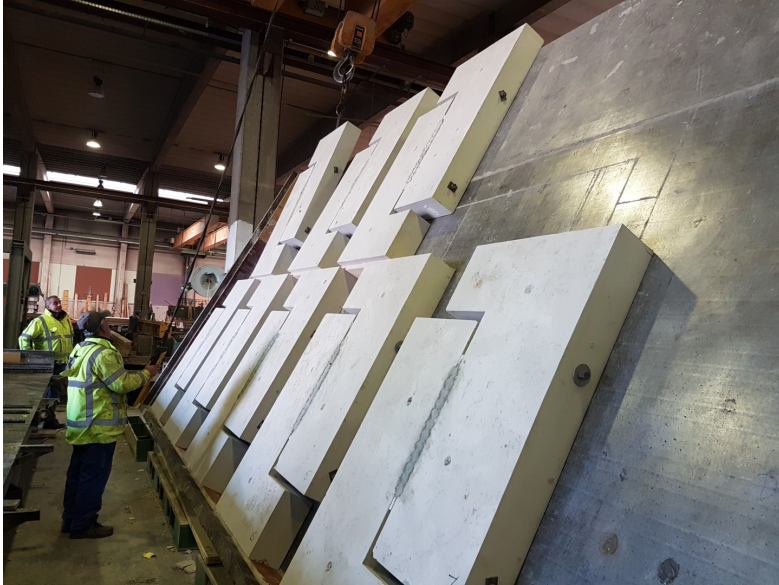
Figure 4.12: Tilting the table just before hoisting the specimens
