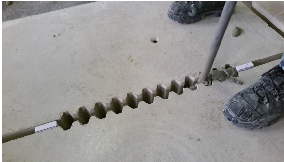
Figure 4.10: Inserting the mortar with a hose
