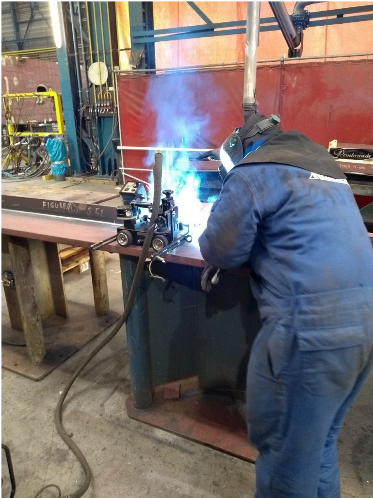
Figure A.5: Welding process in action
