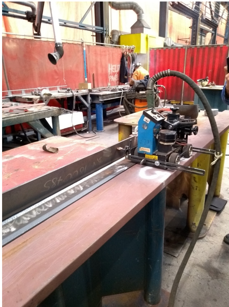
Figure A.4: Use is made of mechanized welding machine for better weld consistency
