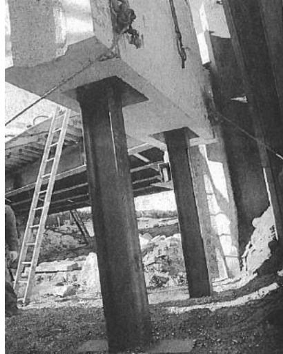
Figure 2.5 - Precast abutment elements with cavities (eventually filled with cast in place concrete. Source: [4]
