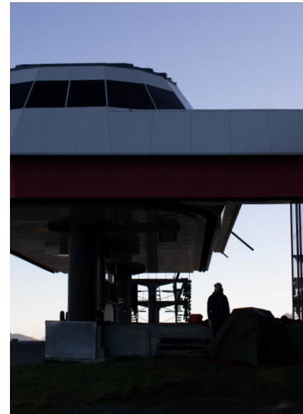
1 st Night: 2048m, Top Station Wartherhorn Express
