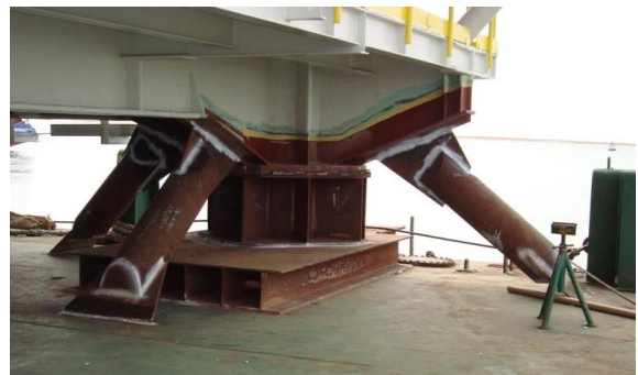
Figure 18: Example of Sea-Fastening
