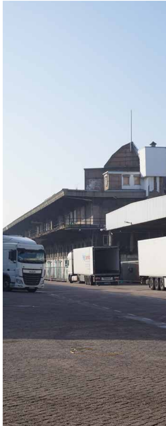
Derelict warehouse in between new activity
