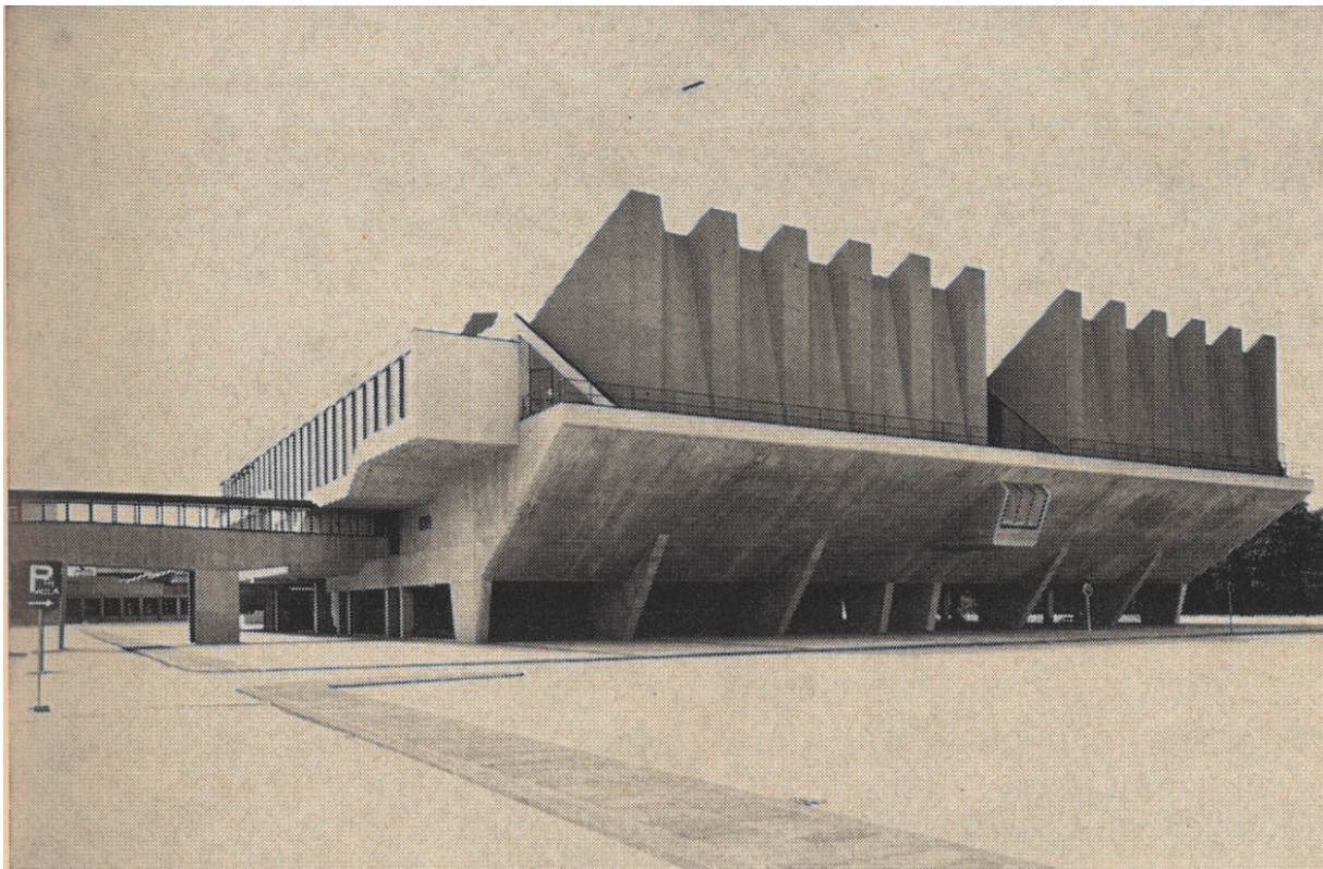
Figure 3.2: Backside of the auditorium (Roelofsma, 1966).
