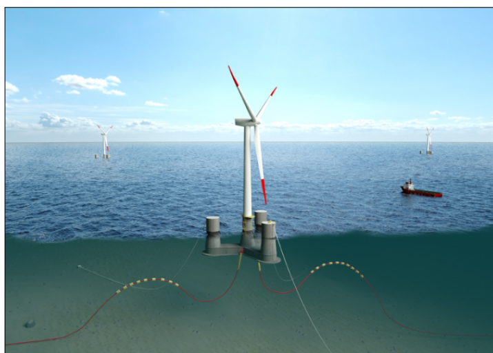
Figure 1.3: DTU 10MW FOWT Mounted on a OO-Star Wind Floater Semi 10MW Floating Substructure [9]
