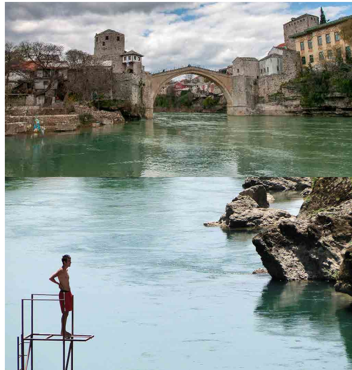
Fig.77 High water level at Old Bridge figure source: https://everything-everywhere.com/unesco-world-heritage-site-236-old-bridge-area-of-the-old-city-of-mostar/
