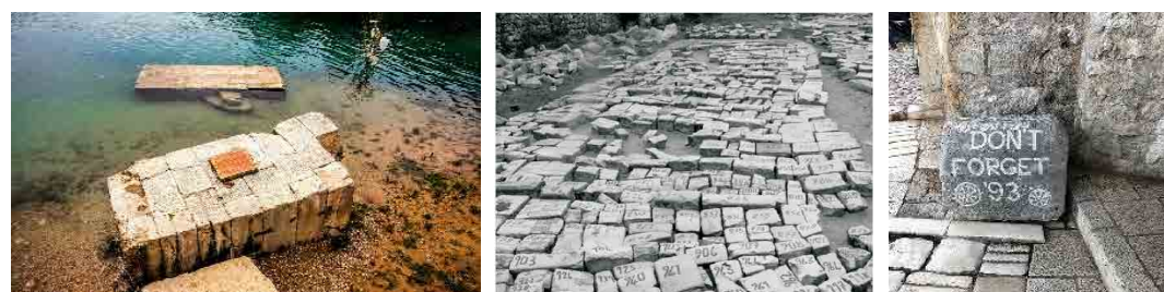
Fig.37 Reuse of original stones for reconstruction of Old Bridge figure from: http://www.cidom.org/ ,
