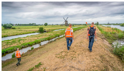
Figure 1.1: Visual dike inspections during drought. [9]
