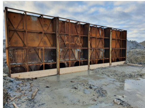
Figure 1.4: Example of an outflow at the Fehmarnbelt project, Denmark
