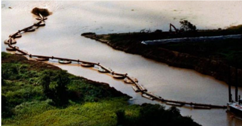
Figure 5-29: Example of pipeline flexibility.
