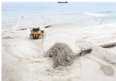
Figure 2-4: Depositing by pipeline.
