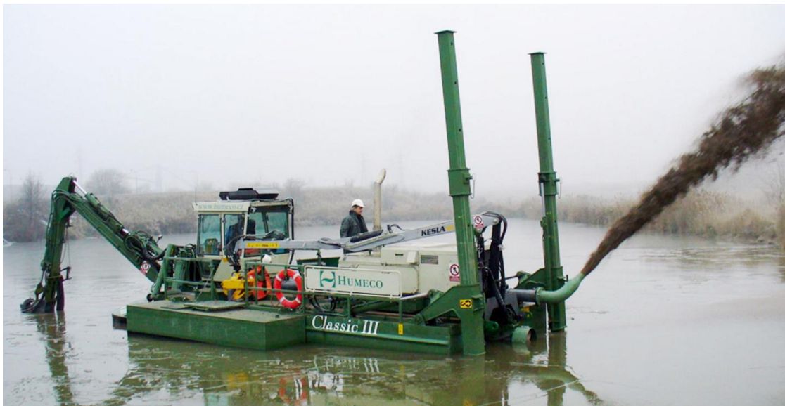
Figure 3-10: Spray pontoon equipped with spuds as propulsion. (Source: dredgingtoday.com )
