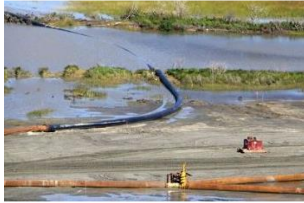
Figure 5-31: Rubber pipeline. (Source: dredgingtoday.com )
