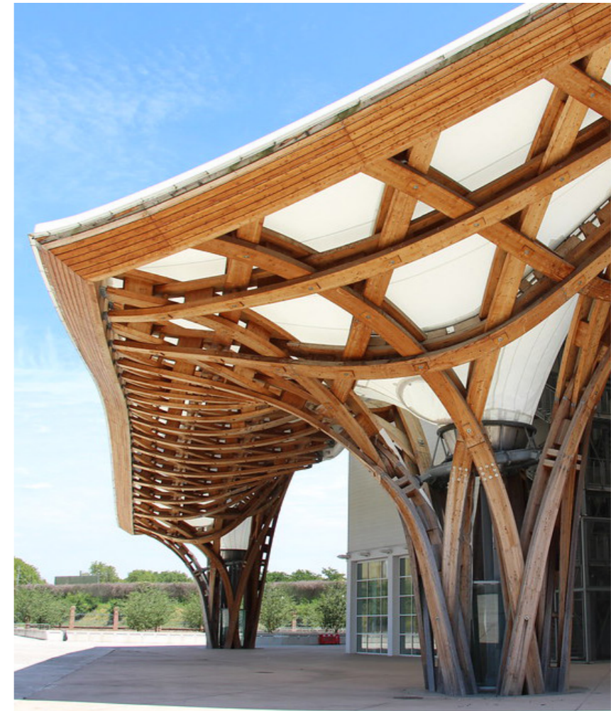
Timber gridshell with semi-regular kagome pattern of the center pompidou in Metz, France.
