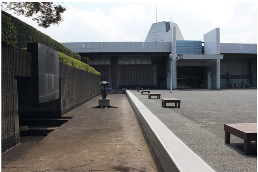
Figure 69 Entrance Area of the Chiba Forest of Culture. © Sumiko Ebara, 2018.
