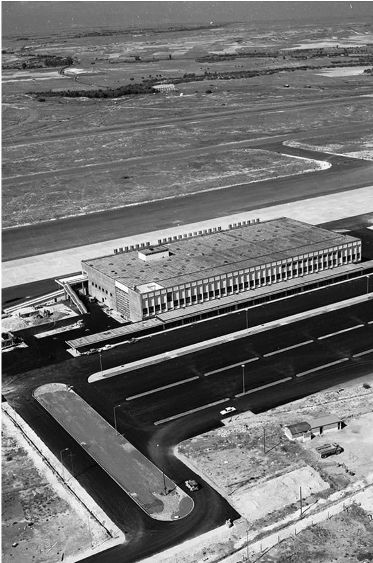
Figure 137. A bird's-eye view of the 1960s terminal building at Nicosia International Airport, taken in 1968. © Press and Information Office, Republic of Cyprus.
