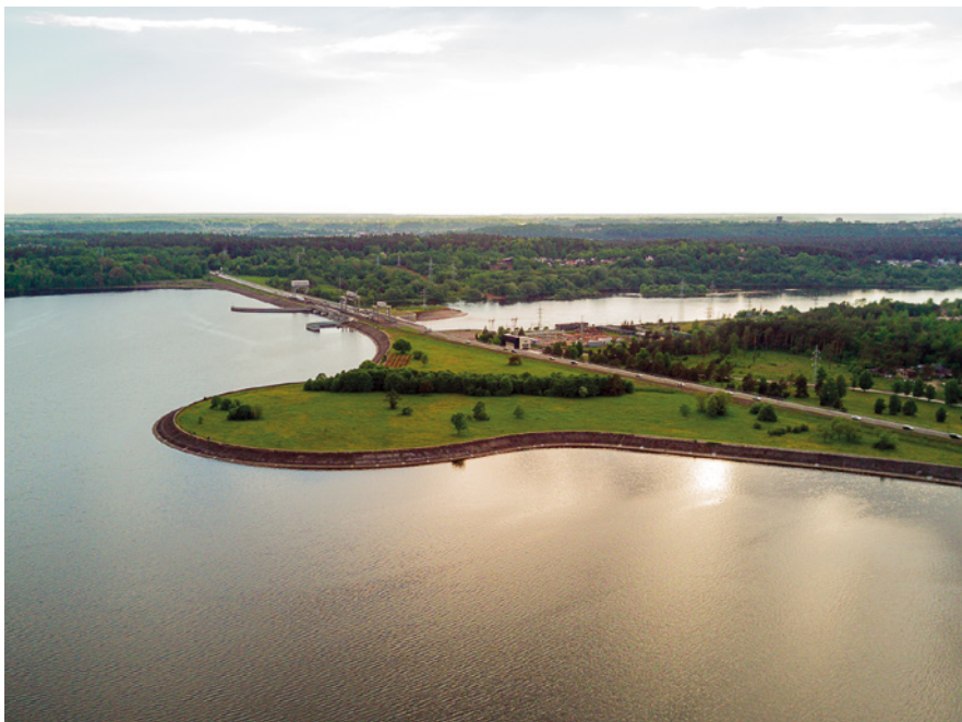
Figure 158 View of Kaunas Hydroelectric Power Plant and its landscape. © Gintaras Gintautas, 2015.
