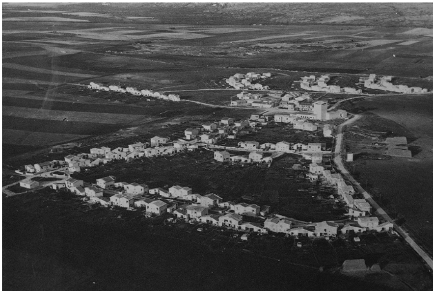
Figure 152 General view of the site of La Martella. © Quaroni Archive.
