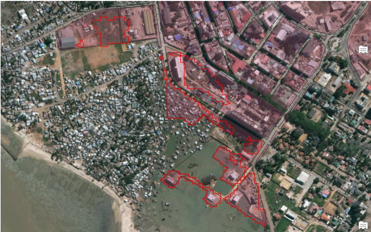
Figure C.4: Aerial pictures of the damaged commercial area in Beira
