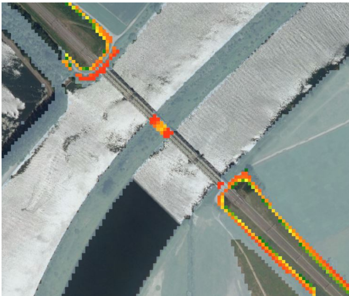
Figure A.12: Calculated Railroad damage at an elevated bridge and elevated berms at a river crossing.
