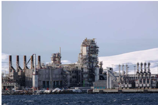
Melkøya gas processing island
