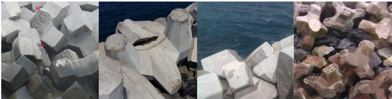
Figure 1: Broken single layer units in reality. From left to right: Xbloc®, Core-loc™, Accropode™, and Accropode™ II (courtesy Royal HaskoningDHV, reprinted from Hofland et al. 2019).
