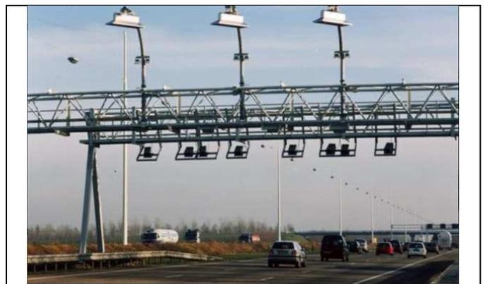
Fig. 1. License plate detection of Camera detection of a road pricing system
