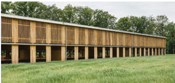
Figure 4-6: Car park Bad Aibling ( B&O Wooden Multi-Storey Car Park, Bad Aibling, n.d. )
