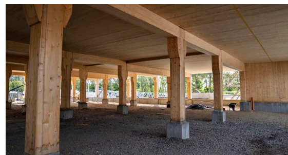
Figure A-20: Load-bearing system Sege Park (Rosholm, 2021)
