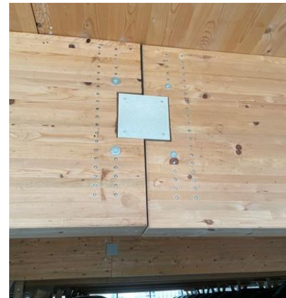
Figure A-13: Connection joist-joist
