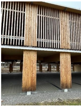
Figure 10-41: Wood protection panel reference project Bad Aibling
