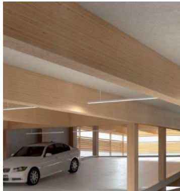
Figure 4-8: Render concept car park of Pollmeier and TUMWood ( Development of Construction System for Multi-Storey Car Parks in BauBuche, n.d. )
