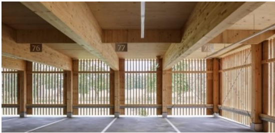
Figure A-30: Load bearing structure of the Bad Aibling car park
