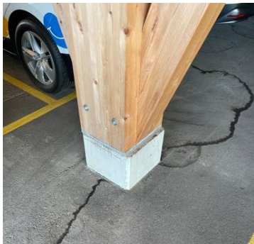
Figure A-8: Column to foundation connection
