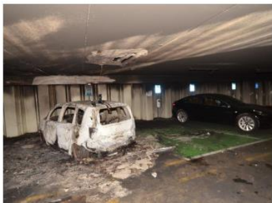
Figure 5-3: Car park fire Alkmaar (Hessels & Ebus, 2020)
