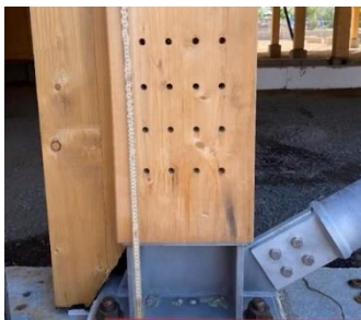
Figure A-23: Column to concrete connection (Plaschke, 2021)
