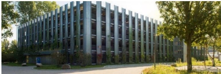
Figure 3-3: ModuPark car park TU Delft P-sports ( Parkeergarage TU Delft P-Sports , n.d.)
