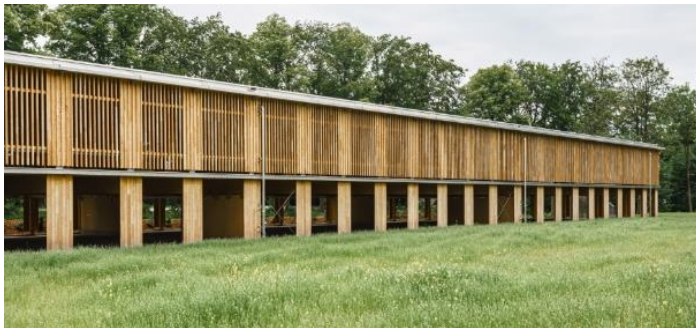
Figure A-26: Car park Bad Aibling Germany ( B&O Wooden Multi-Storey Car Park, Bad Aibling, n.d.)
