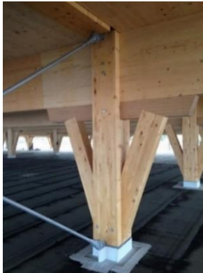
Figure A-16: Connection pillar to beam (Zaugg, 2018)
