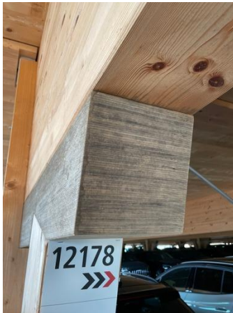
Figure A-12: LVL beam first level
