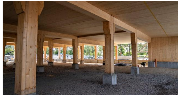
Figure 4-5: Load-bearing system Sege Park Malmö (Rosholm, 2021)
