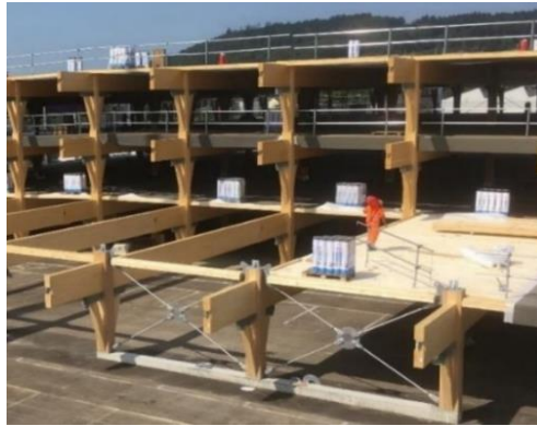
Figure A-17: Erection CLT floor (Zaugg, 2018)
