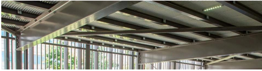
Figure 6-12: Construction Park4all FRP floor system (Park4all - Parking Solutions, n.d.)
