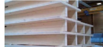
Figure 6-16: Timber composite floor KLH ( Rib Elements, 2019 )
