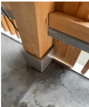
Figure A-28: Column protection first level
