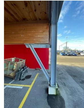
Figure A-18: Façade column to joist connection
