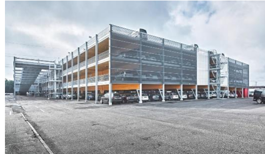
Figure A-7: Car park façade Studen (Zaugg, 2018)
